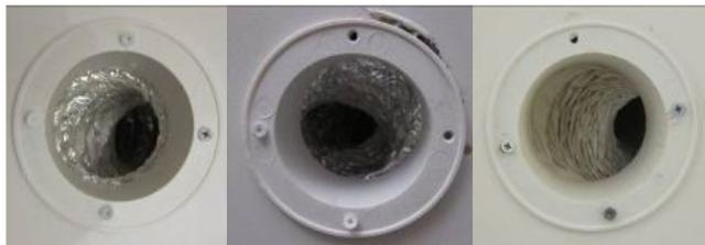
Figure 4-57 Extract terminals with diffusers removed showing constrictions in flexible ducting.
