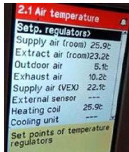
Figure 4-59 Photo of an AHU display that shows temperature measurements in the supply and exhaust.
