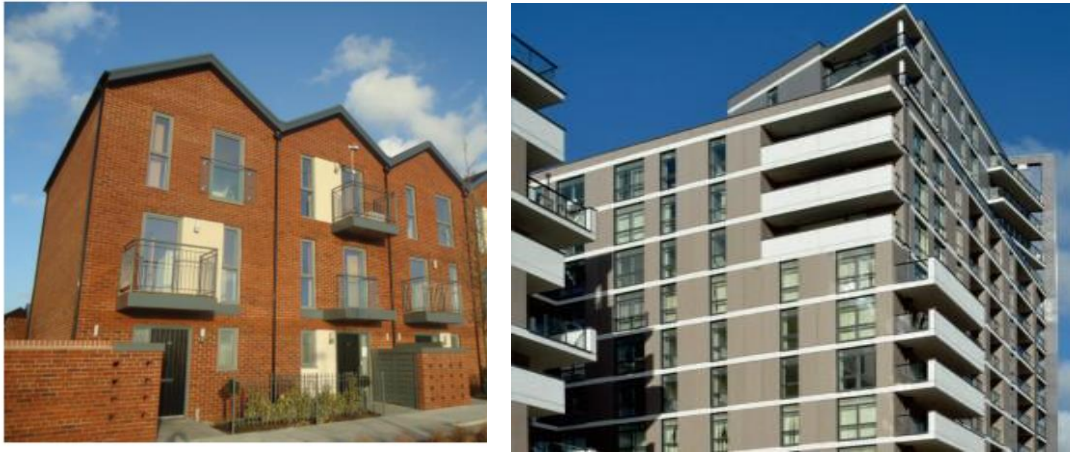
Figure 1: Examples of dwellings covered in the study: terraced houses with MEV system (left), apartments with MVHR system (right)
